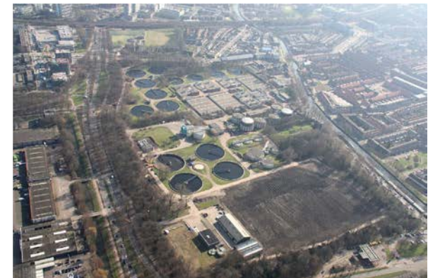
Water sewage plant RWZI, Utrecht
